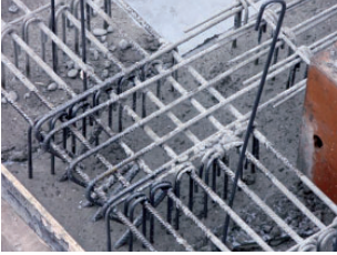
Figure 3.5 - Ancrages courbes
