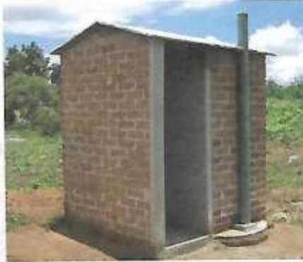
Figure B : latrine
