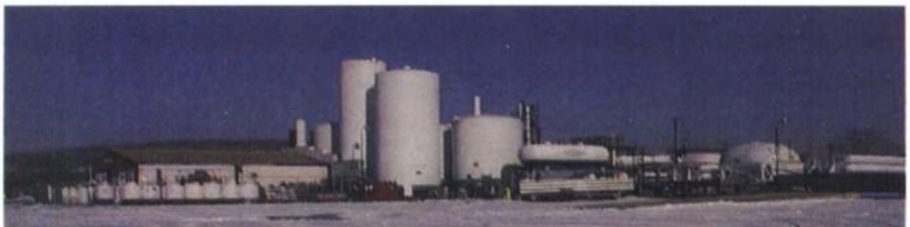
Manufacture of Hydrocarbon refrigerants.
